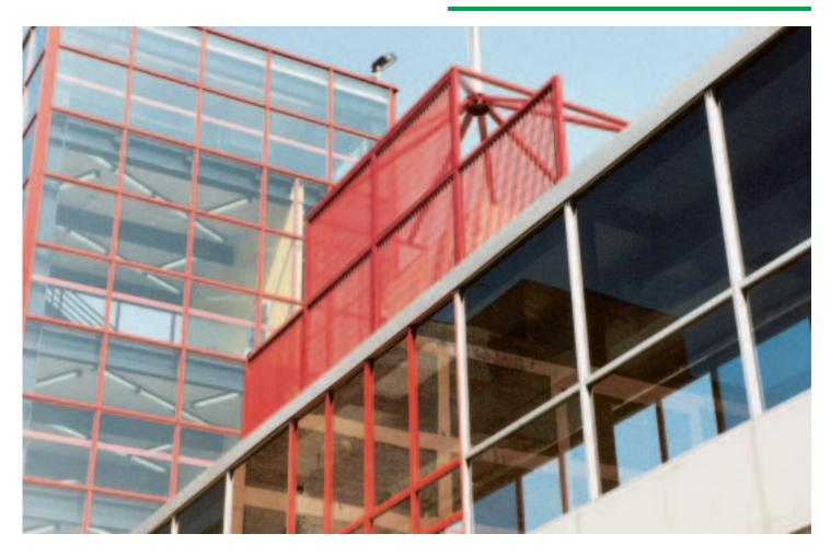
Ametco grilles are manufactured from electro-forge welded steel giving you the strength required for security. Ametco can custom fabricate any of the standard meshes to fit your needs. All grilles are hot dip galvanized after fabrication then powder coated. This combination not only gives you the best protection but also allows you to choose a color from Ametco's 15 standard colors to harmonize with the surrounding environment.
