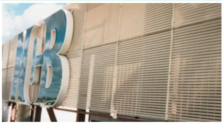
Ametco Mfg. Corp. has the industry's largest selection of architectural grilles and screens. From electro-forge welded steel grilles to extruded aluminum louvers; Ametco can work with you to achieve the requirements of your project. All of Ametco's grilles and screens are polyester powder coated to any of the 15 standard Ametco colors.
